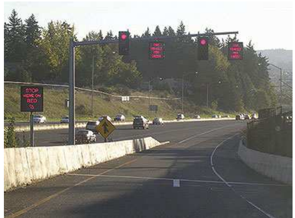
Figure 8: The expressway self-throttles its traffic by limiting the number of entering vehicles. Drivers often ignore this red light thus overriding the expressway's setting.
